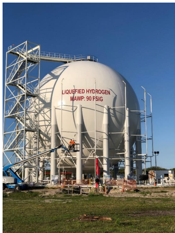
Figure 34: World's largest liquid hydrogen storage tank under construction Source: Swanger [61]
