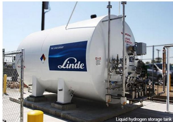
Figure 33: Above-ground, LH 2 tank Source: Hydrogen Fuel Cell Partnership [60]
