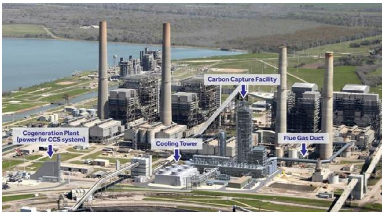
Figure 2: Petra Nova coal-fired power plant with CCS system, near Houston, Texas Source: U.S. Energy Information Administration [5]
